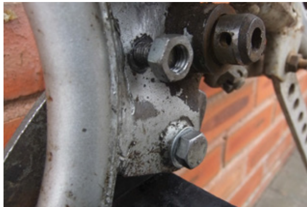
10. Photo shows the bolts from rear of the frame
